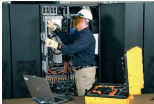
Quelle: Eaton Power Quality
